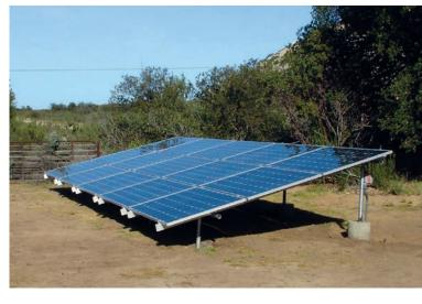
A ground-mounted 4.125 kW batteryless PV array—15 SolarWorld 275 W modules and 15 Enphase M250 microinverters—provides the home's energy generation. This array was sized to meet the anticipated needs of this all-electric home but has proven to be larger than needed. An electric car could easily be charged with the surplus electricity. Once energy-storage prices drop, a battery bank would be an asset to this remote rural home when the grid goes down.
