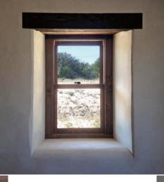
Above: Besides providing good insulation, the two-foot-thick strawbale walls lend themselves to sculptural interpretation, especially around window openings. The flared window shapes in this home echo the window shapes at local historic ranchos (left) and missions (right). This technique minimizes glare by creating a light gradient from the bright outdoors to the more subdued indoors.
