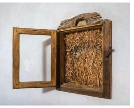
A truth window is a small opening in the wall that reveals the substrate behind the plaster—strawclay (above) and straw bales (below). A tradition in strawbale houses, truth windows are a source of surprise and delight as guests get a peek inside.
